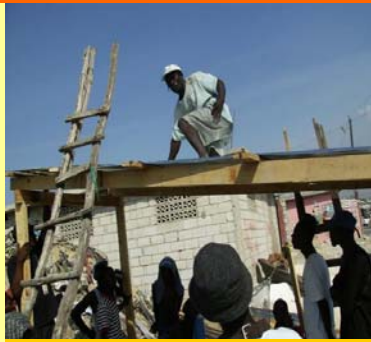
Building tin roof shelters to house displaced persons
